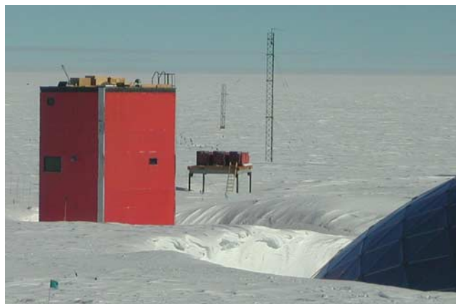
Figure 8. South Pole neutron monitor environment. Skylab is prominent structure at left; neutron monitor is on platform to right of Skylab; the edge of Dome is far right. Since 1977 the neutron monitor has been raised a total of 18 feet to keep it above the surface of the snow. As surrounding structures are buried, this changes the environment and potentially has a systematic influence on the count rate.
