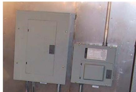
**Resistance Heaters.** Located on both sides of the TasVan. Power is controlled by the circuit breaker for the 220-volt service. Turning this breaker “off” disconnects power to the unit. The resistance heaters are used only in Antarctic waters. They are secured during the passage from Seattle to Sydney and on the return passage from Adelaide to Seattle. Thermostatic controls for these heaters are located on the heaters.
